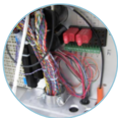
Figure 8: OSP Connections at the DSLAM
