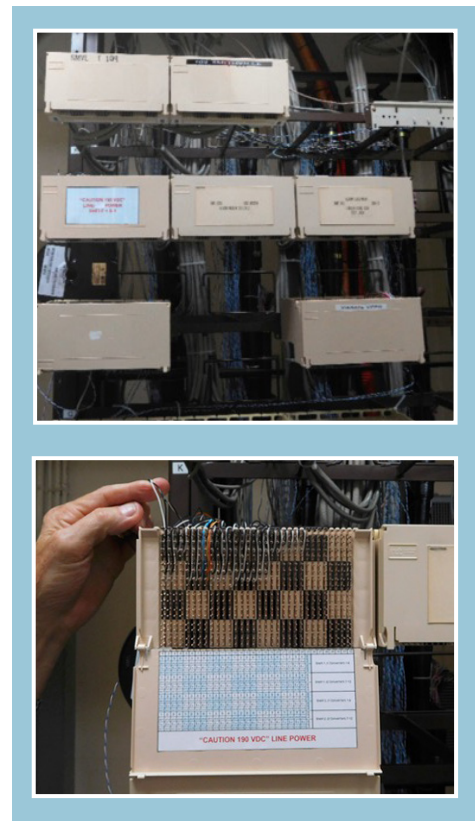
Figure 3: Horizontal Connector with Precautionary Labels
