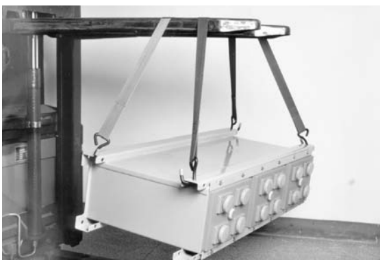
Figure 5: Positioning the module onto the base channels
