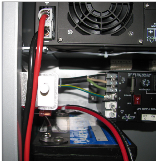
Figure 7 — Main Harness Routing
