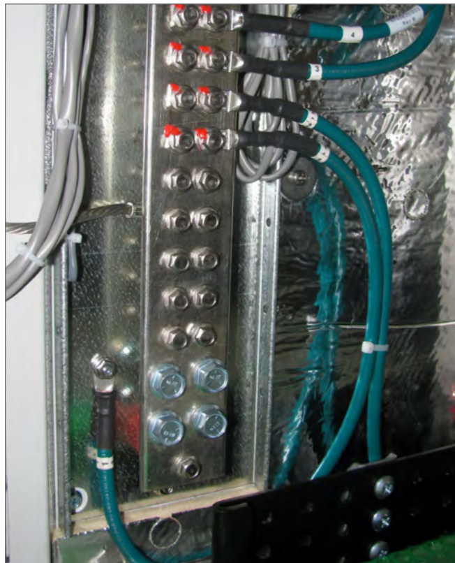
Figure 6 — Enclosure MGB and Chassis Ground
